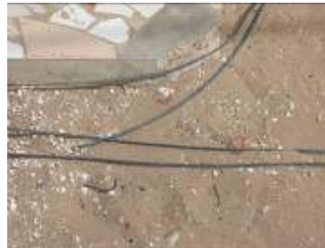
Undersized connections
